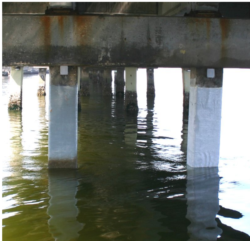
Figure 5.15 Piles after FRP repair with UV coating.
