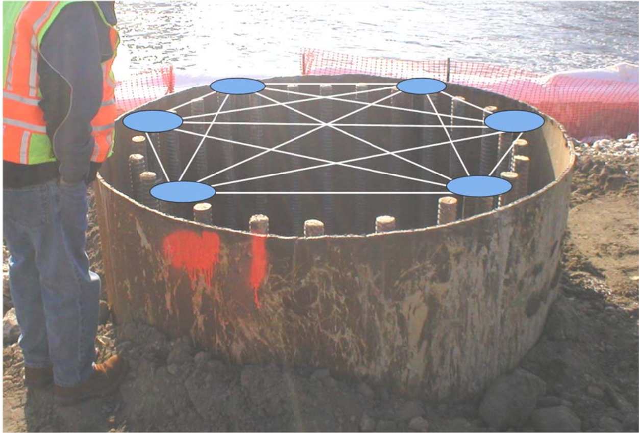
Figure 3.3 Testing coverage from acoustic (lines) and gamma radiation (circles) methods.
