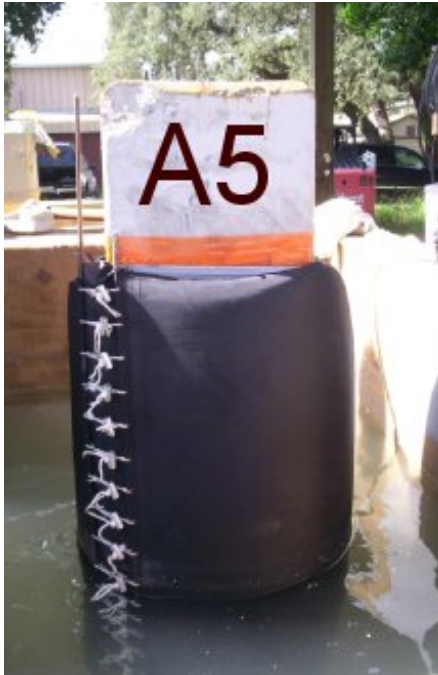
Figure 5.9 Pressure bag applied to pre-preg system.
